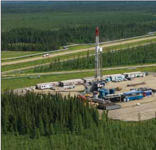
A drilling site at Christina Lake.
