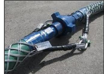
(Acceptable pipe restraints systems for temporary piping)
